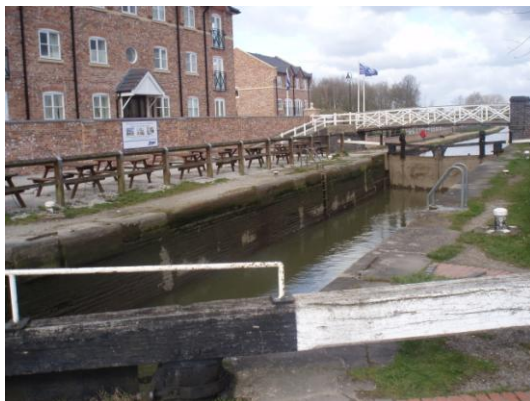
O – Middlewich Lock
